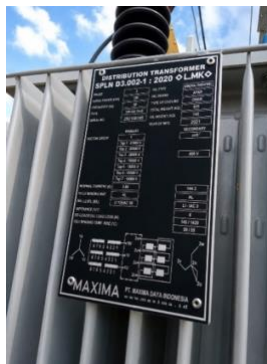
Gambar 2. Nameplate Transformator
